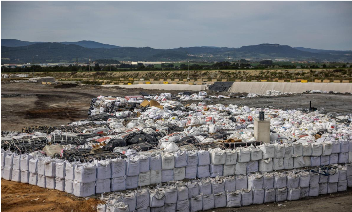
Image 2. Disposal in an authorized landfill of asbestos-containing waste under the traditional prolonged confinement model.
