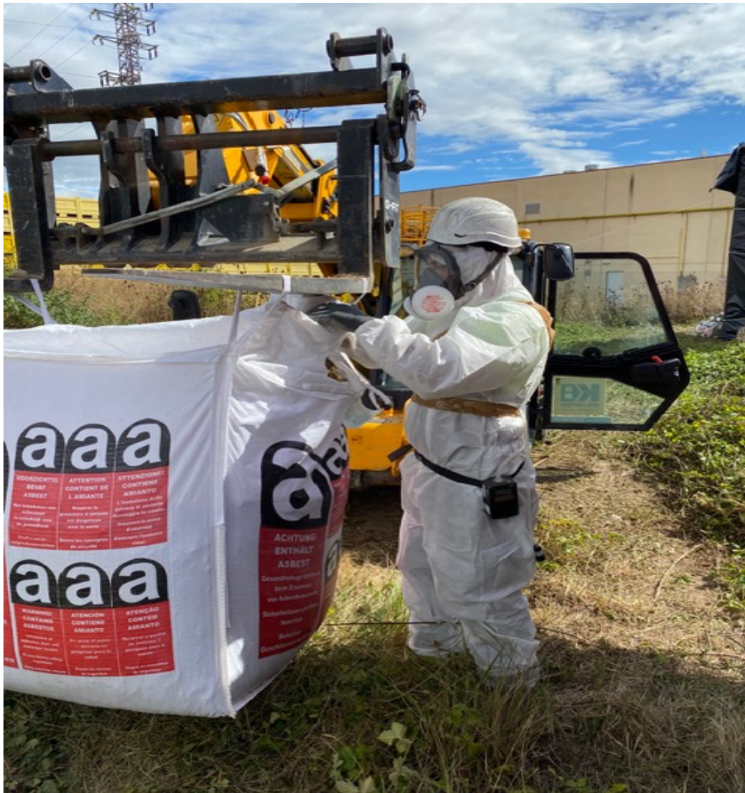
Image 3. Handling and temporary storage of asbestos-containing waste in approved big bags under established safety protocol.
