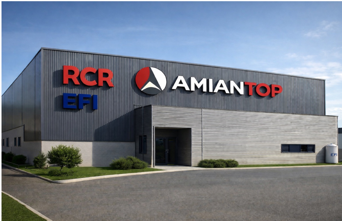
Image 5. AMIANTOP industrial infrastructure – Base configuration with FS GREEN® technology (9,8 t/day).
