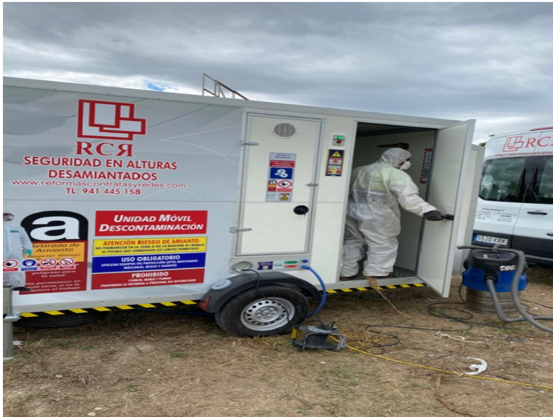
Image 4. Mobile decontamination and logistical support unit devduring controlled asbestos removal operations.
